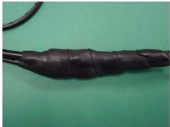
10) Apply three overlapping layers of PVC electrical tape, extending 1" beyond the previous layer with each wrap.
