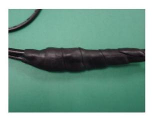
10) Apply three overlapping layers of PVC electrical tape, extending 1" beyond the previous layer with each wrap.
